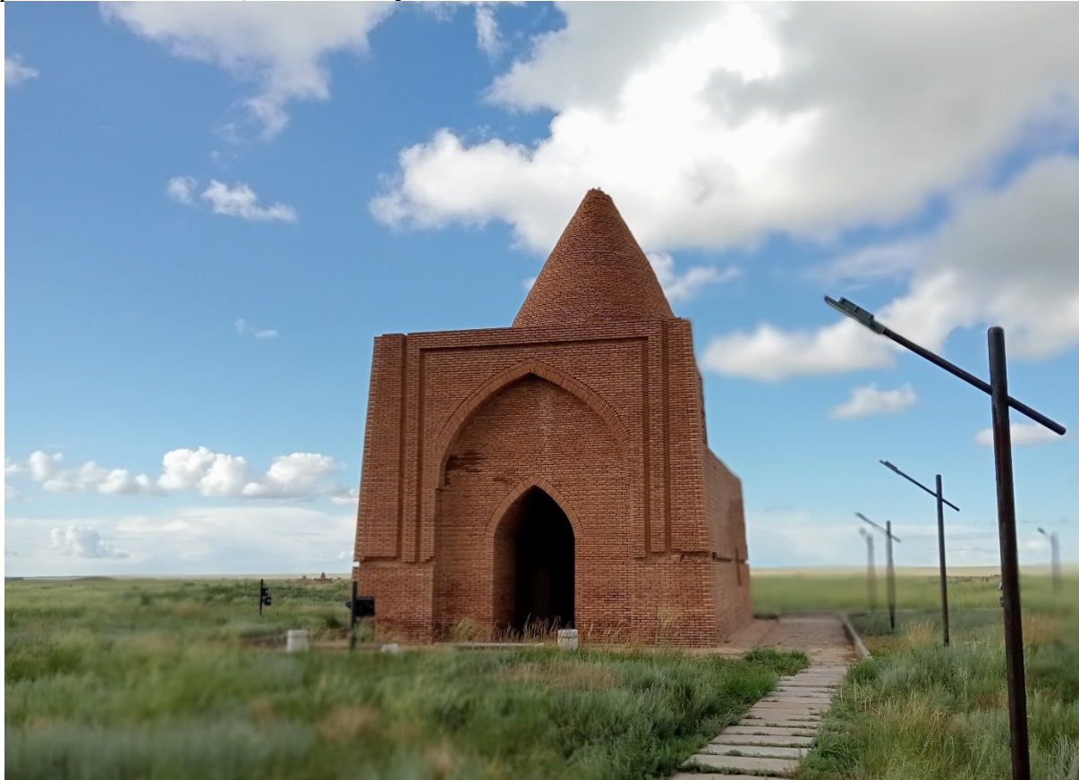
Fig. 2. Abat-Baytak mausoleum after restoration.
