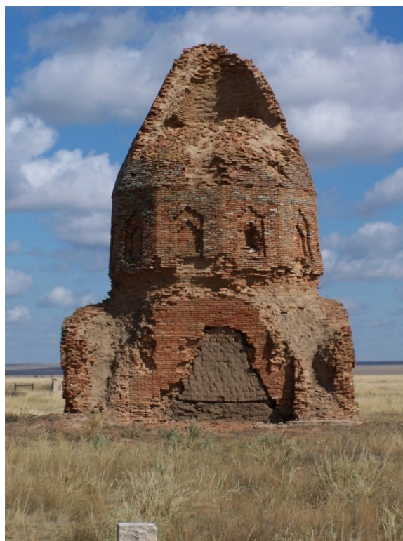
Fig. 1. Abat-Baytak mausoleum before restoration. Photograph from the collections of the Centre for Preservation, Research and Restoration of the Aktobe Region Department of Culture.
